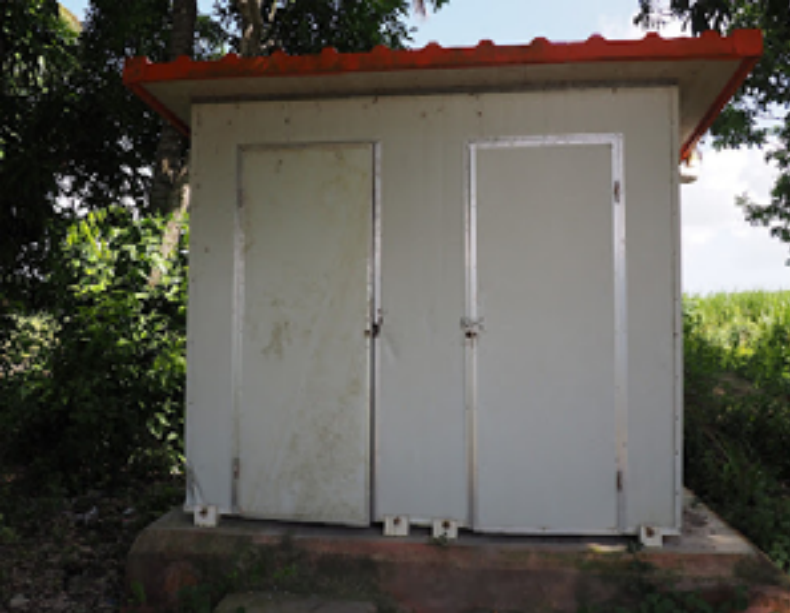
The replaced exterior of a latrine in Batey Bermejo in July 2024.
