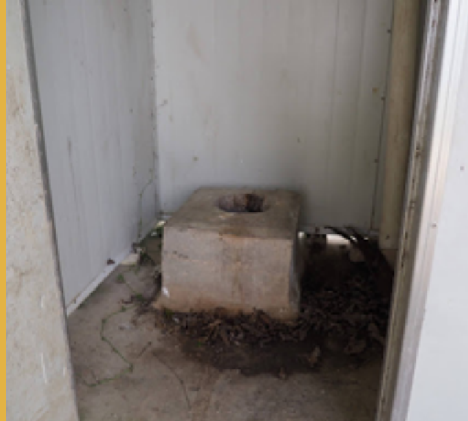
The interior of that same latrine, which appears identical to the interiors of the old latrines.
